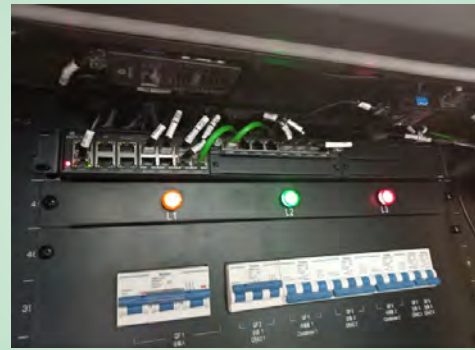
30 KVA dedicated Generator and Vertiv Power Distribution Unit
